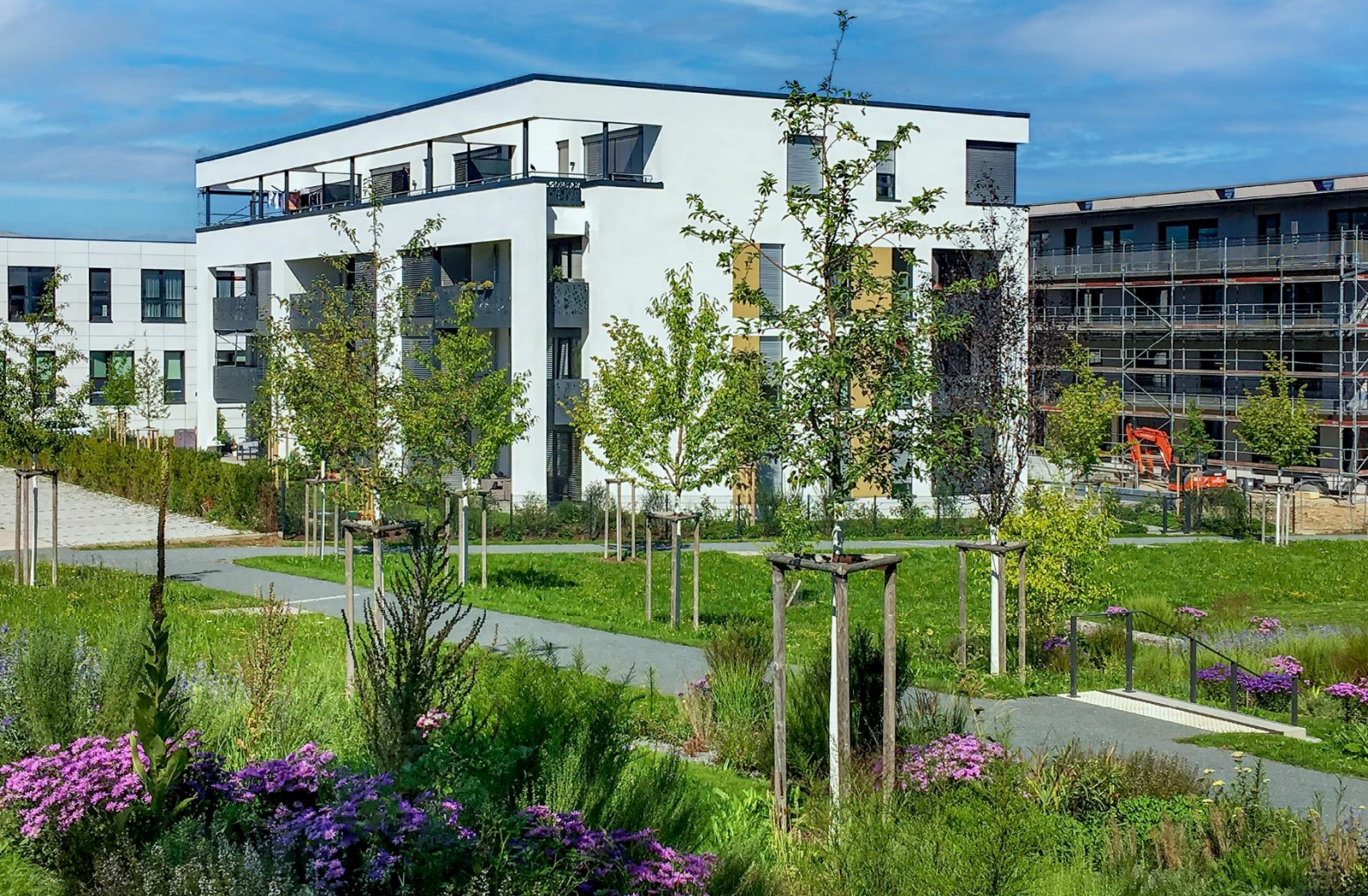
Am Terrassenpark multi-storey apartment block, Würzburg Income-based subsidies Builder-owner: Ruth, Sabine und Daniela Reinfurt GbR, Würzburg Planner: Grübel Architekten, Neu-Isenburg Photo: Government of Lower Franconia, Würzburg
