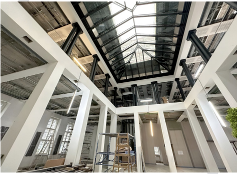
Construction site with a view through the roof
