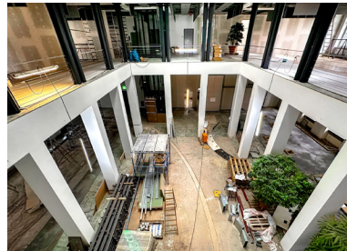
Construction site on the ground floor
