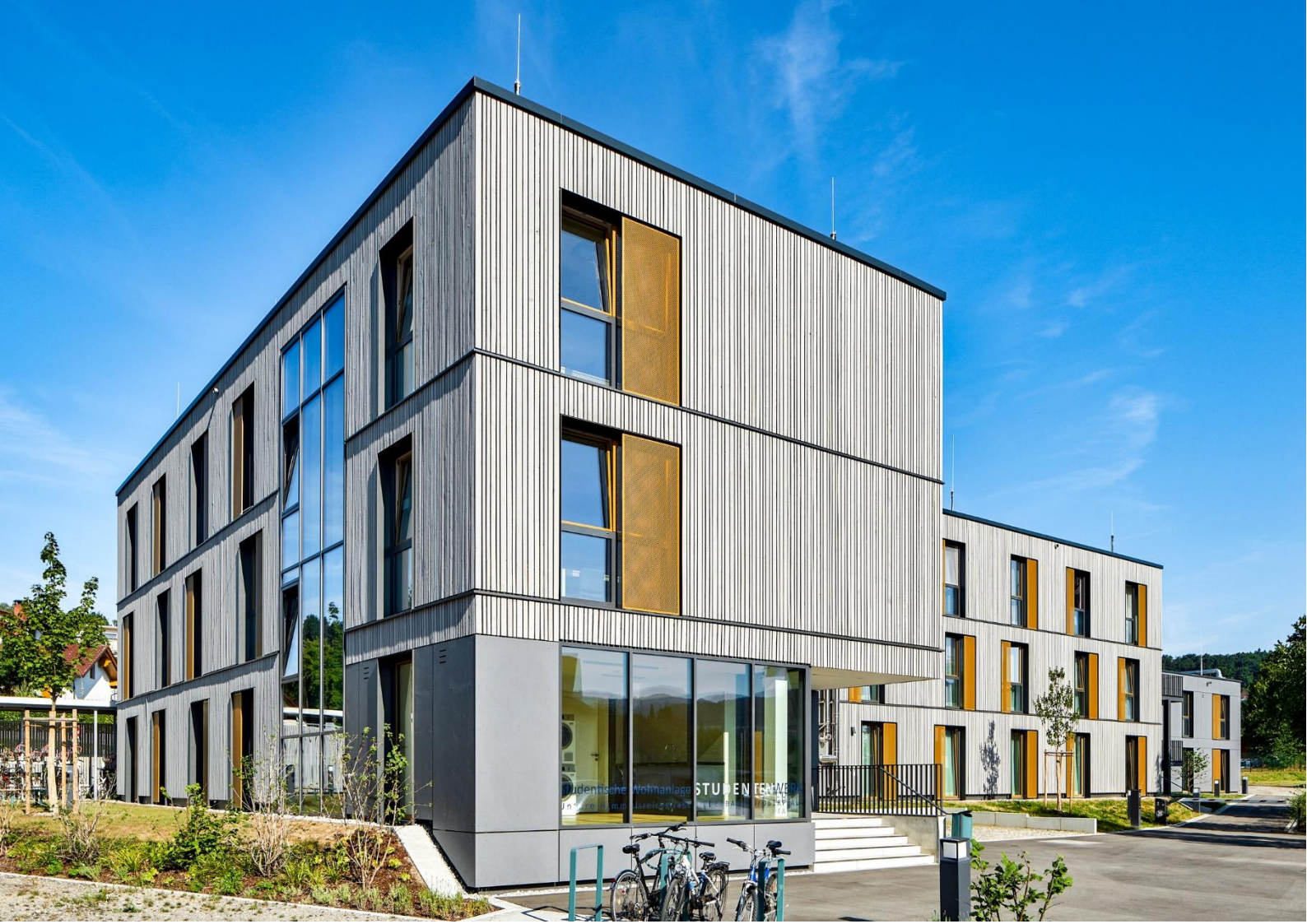
Deggendorf student residence Subsidies for student accommodation Builder-owner: Studentenwerk Niederbayern/Oberpfalz Planner: karlundp Gesellschaft von Architekten mbH, Munich Photo: Connolly Weber Photography GbR, Munich
